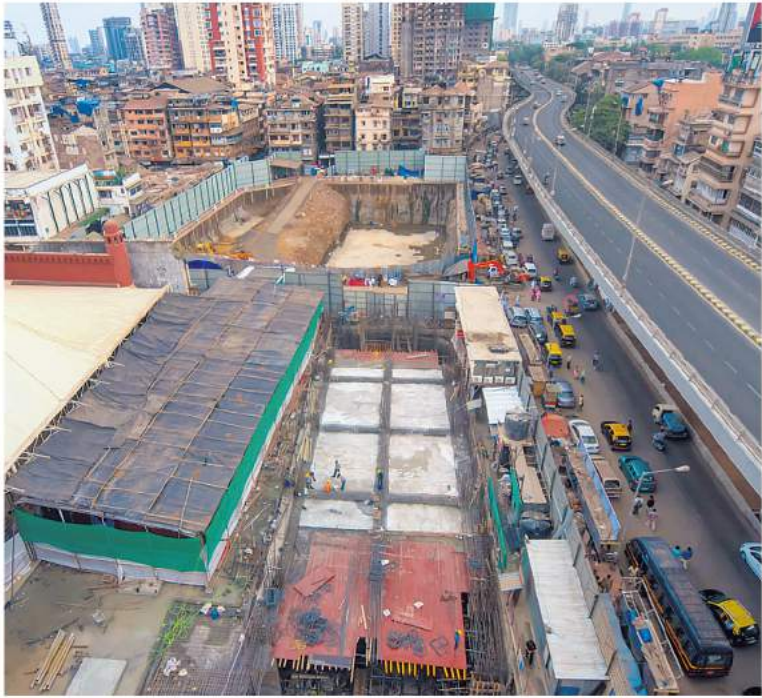
The Bhendi Bazaar redevelopment, phase 1 and 3 is currently on
